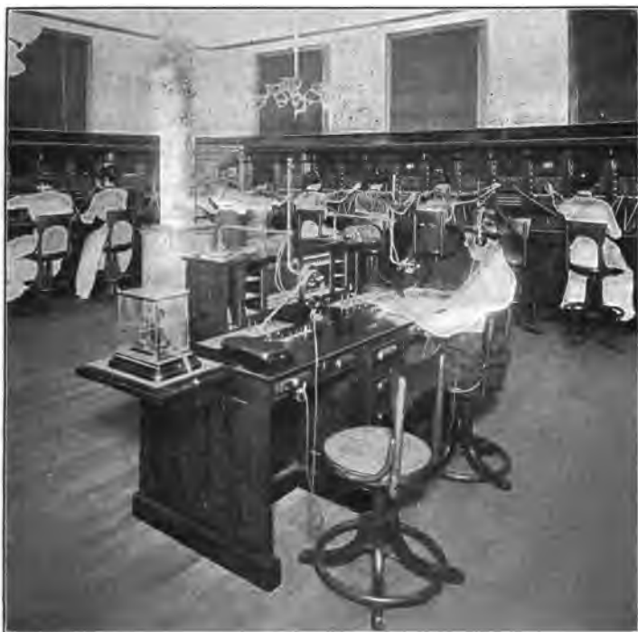
FIG. 94.—Operating Room in a Small City Exchange.
